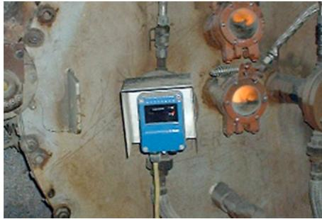
For high-temperature applications, such as cyclone boilers, we designed the 16283 Hi-Temp Accu-Flame Sensor. When used with optional heat shield and thermal barrier, it is able to withstand the toughest applications, where other sensors fail. An integrated LED display allows for simple setup, as well as quick reference of flame quality readings.
